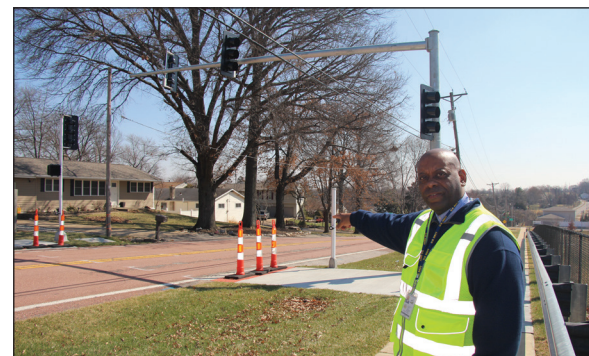
Safety and Security Coordinator Terrell Baker shows off the new crosswalk being installed at Dressel Elementary School.
